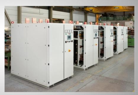
High power **dual** output rectifiers Capacity: 2 x 45 V/ 7,500 A
